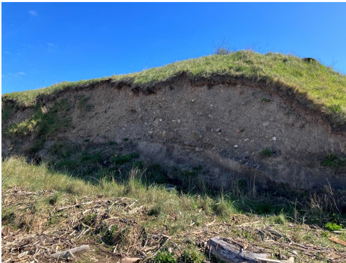
Plate 17A-13: Eroded Edge Of Made Ground At Bran Sands. Note Clearly Imported Material Raising Height Of The Area Of Former Coastal Sands
