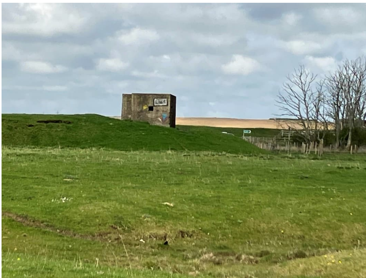
Plate 17A-10: Small, Square Pillbox At Northern Extent Of Former Railway Embankment, Facing North-East
